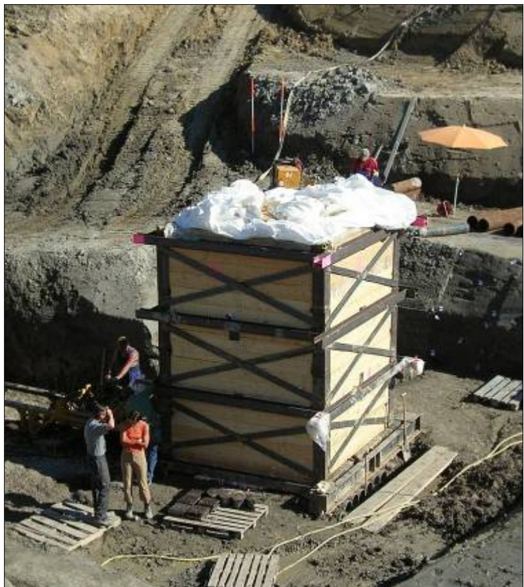
Fig. 1: The block containing the lower three meters of the well shortly before lifting
